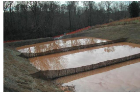
Sediment Basin with Silt Fence Filtration
